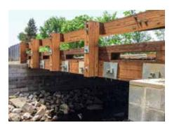
The Geosynthetic Reinforced Soil-Integrated Bridge System provides durability and decreases bridge construction time and cost due to the simplicity in design and accessibility of necessary materials and equipment.
